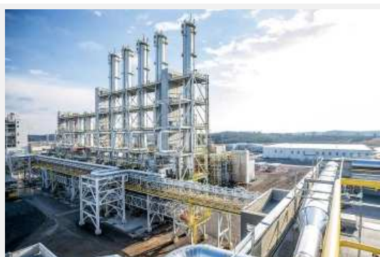
Wacker spent $2.5 billion building this polysilicon plant. Credit: Wacker
