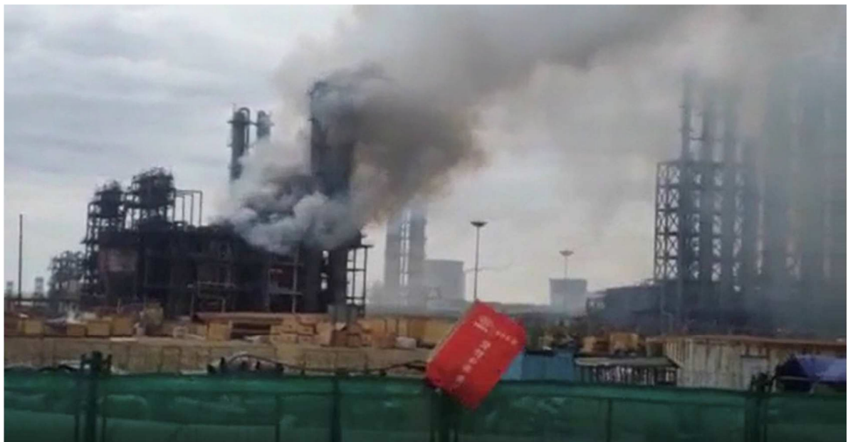
The leakage of a superheater caused a fire at East Hope's polysilicon plant in Xinjiang on June 17 – Screenshot: Bernreuter Research
